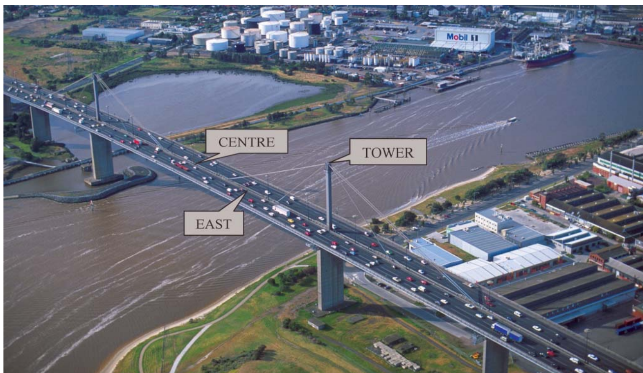
Figure 2: Location of GPS receivers on West Gate Bridge
