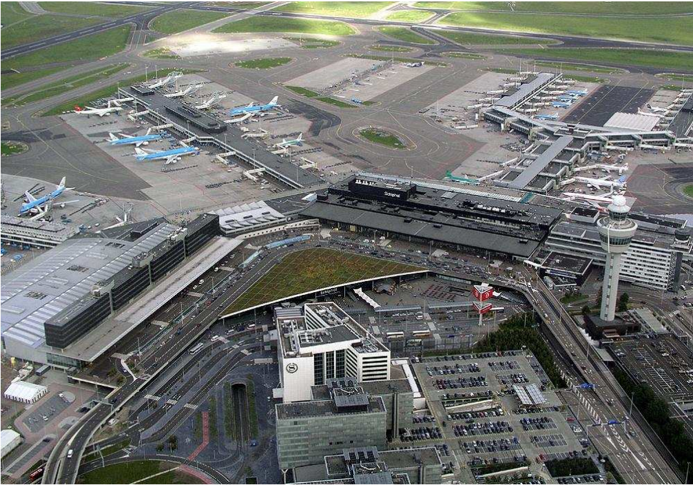
Figure 6. Aerial view of Schiphol Center.
